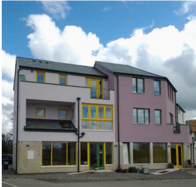
West side - exposed
