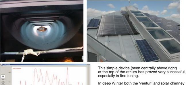
In deep Winter both the 'venturi' and solar chimney are closed down fully . In the shoulder seasons of Spring / Autumn this solar chimney is gradually utilised more or less as required and only in high Summer the Venturi ventilator (see below ) is introduced.
